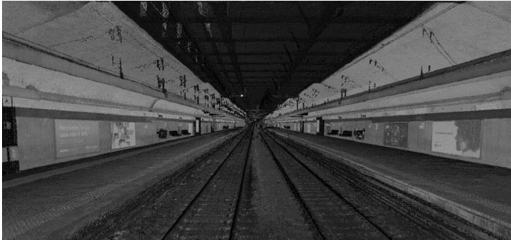
Figure 3: Point Cloud of Metro Station in 3DReshaper.
