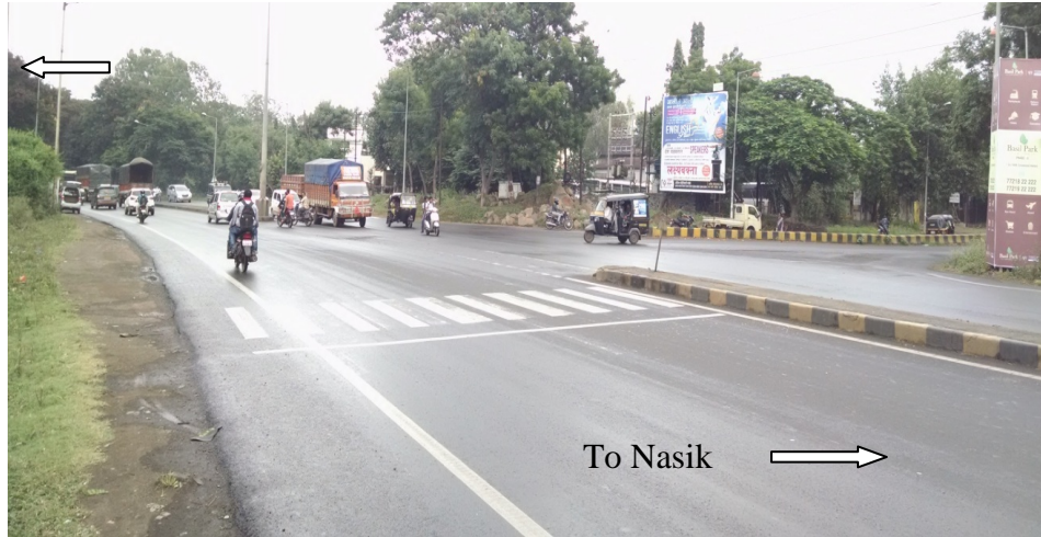
Figure 5: Snapshot showing MIDC Intersection Pune-Nasik Hwy, Pune
